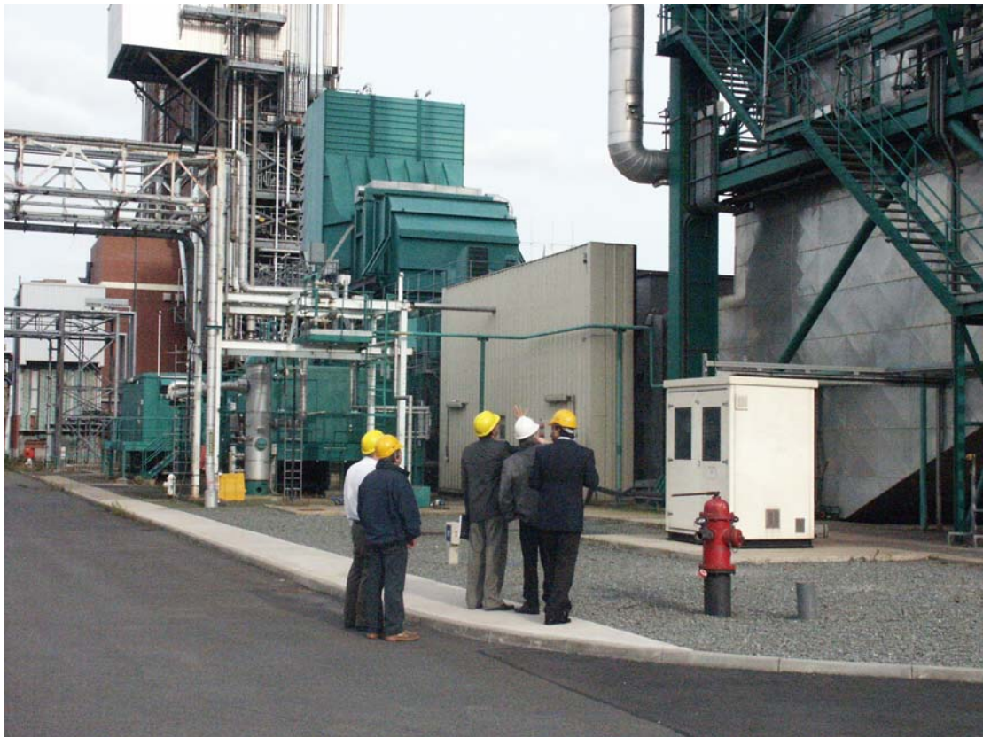
CESS accompany Indian delegation during inspection of 124 Mw Frame 6FA CCGT plant at Cardenden in Fife (Scotland)
